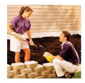
To remove outside lugs or edges of retaining lip, hold unit securely or place at angle on ground. Srike the lug firmly with a hammer. Always wear safety glasses to protect eyes from chips.
